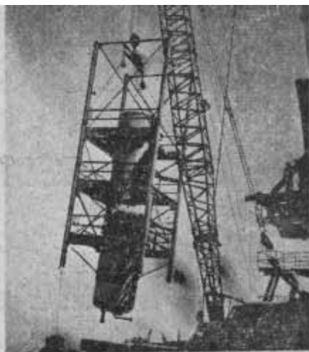
THE BIG LIFT — A 45-ton crane heists the Redstone propellant tank cage into a vertical position at the 500 K. Workmen welded the Redstone modification onto the stand to enable the Redstone missile motors to be tested at the stand. The cage and fuel tanks weigh an estimated 30 tons.
